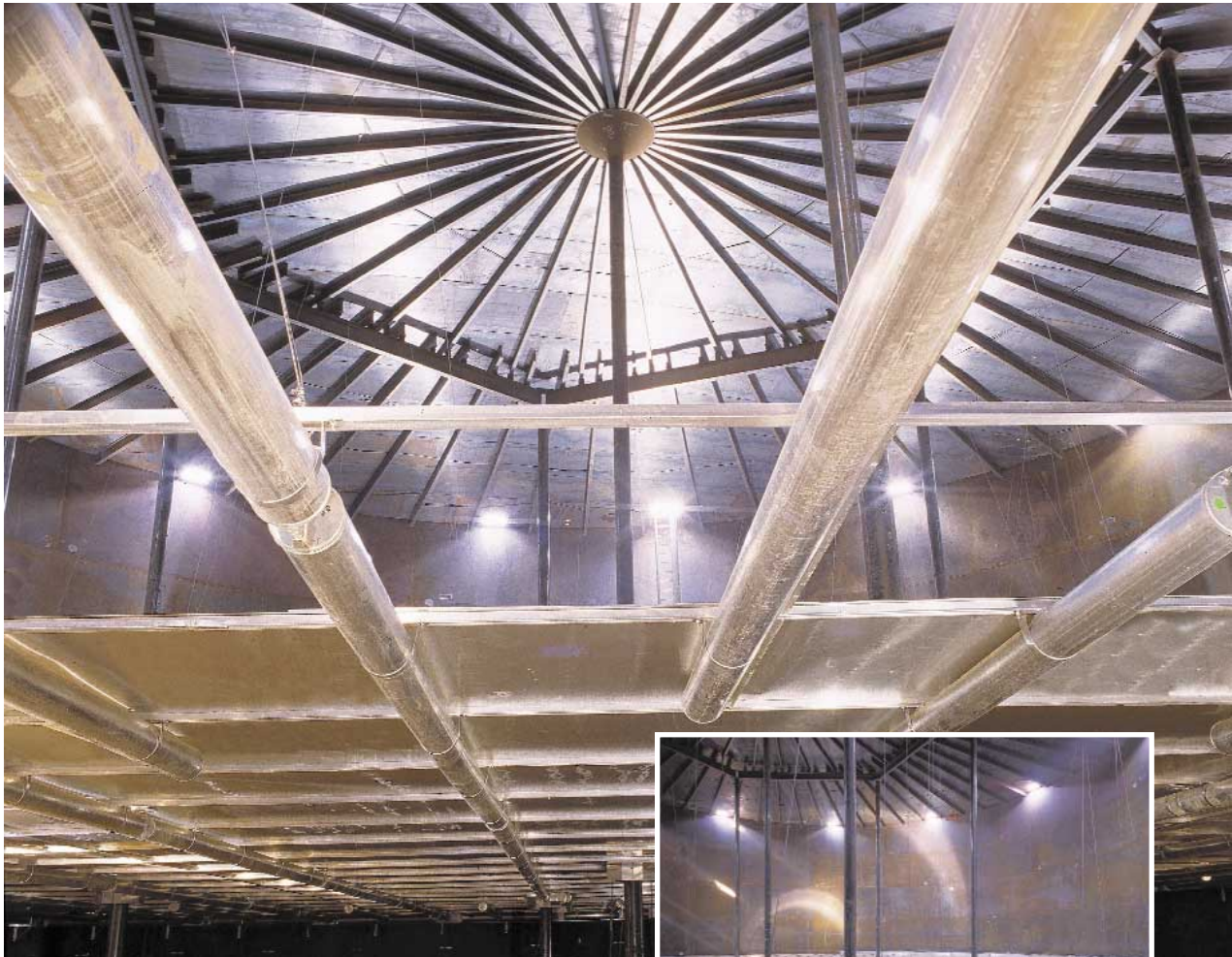
Underside view of pontoon type IFR
