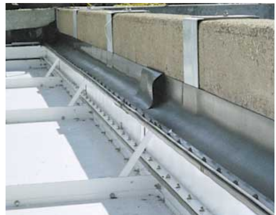
Double perimeter wiper seals.
