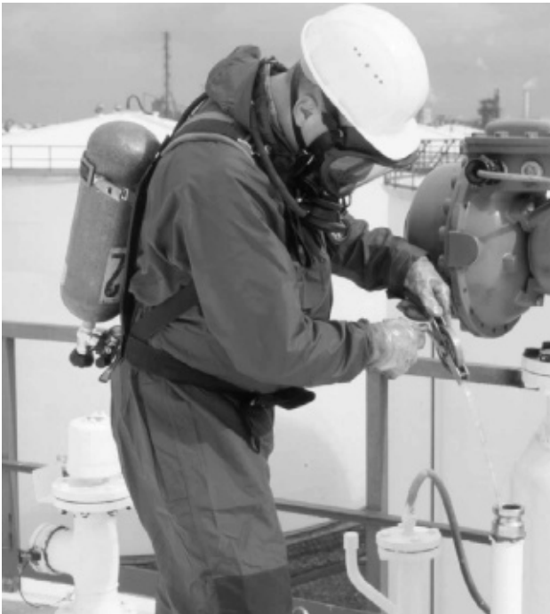
Fig. 5. Manual Gauging
