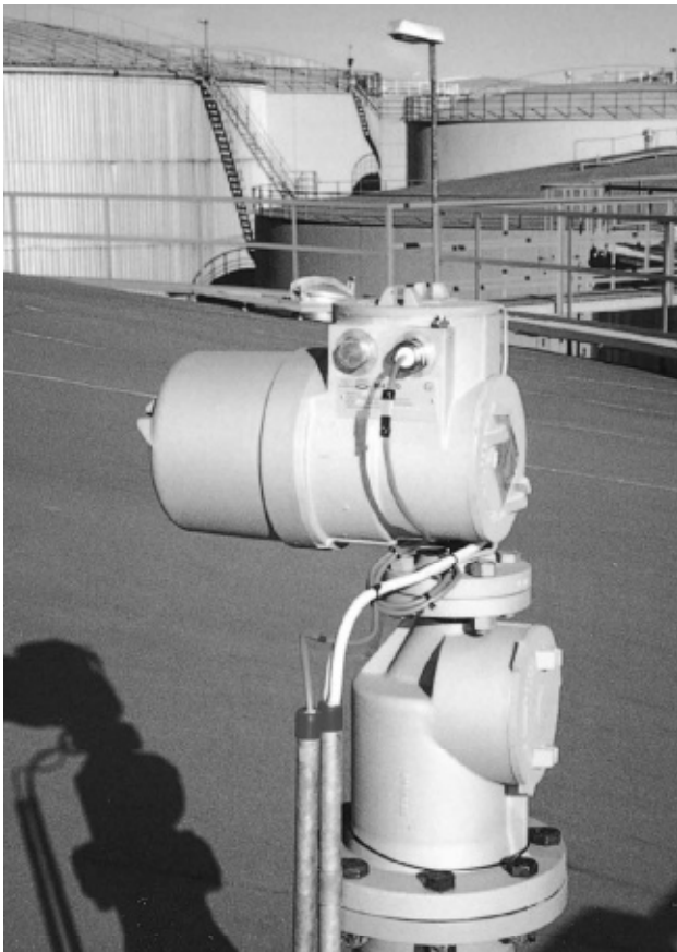
Fig. 7. Servo gauge
